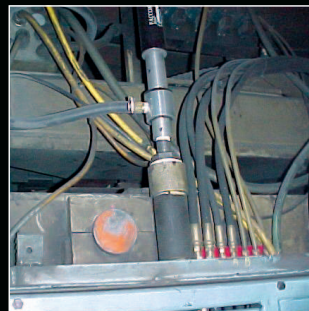
Foundry application: VDF pump solves maintenance problem
